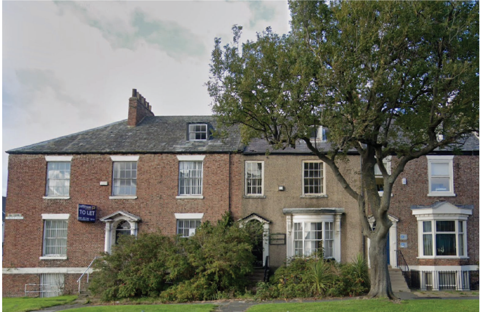
View of Grade II Listed 1 and 3 Beach Road
